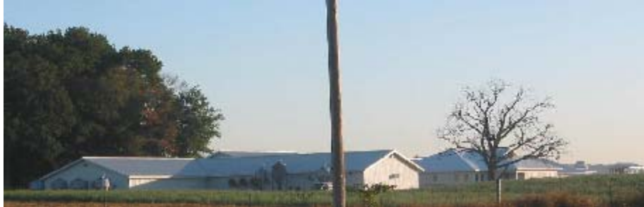
Figure 2 . Le « Swine Research Facility » du Michigan State University
