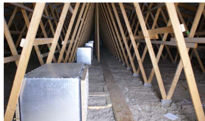
Figure 18 Filter ducts installed in an attic with trusses 48" apart
