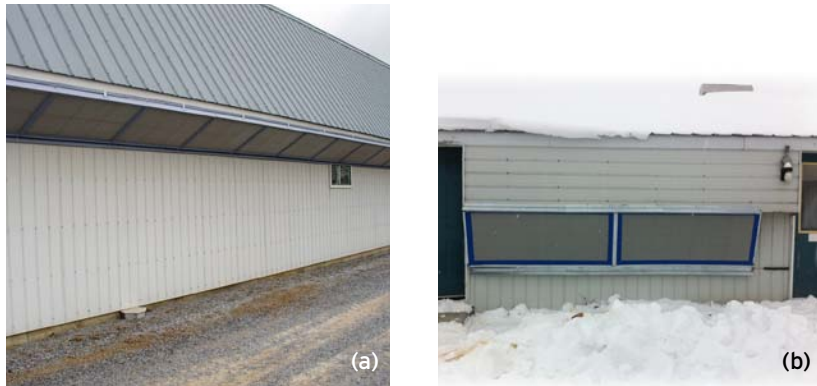
Figure 14 First-generation antimicrobial filters (a) and new generation of antimicrobial curtain filters (b)
