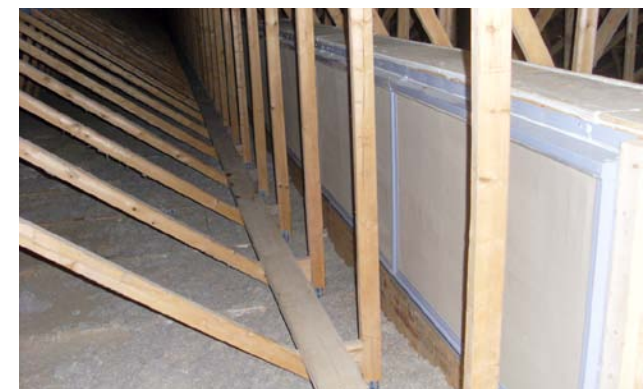
Figure 23 First-generation antimicrobial filter installed on a continuous linear air inlet
