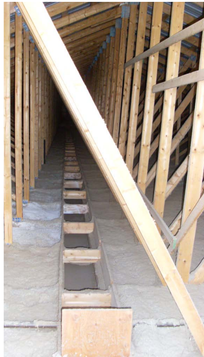
Figure 20 Continuous linear air inlet without filter
