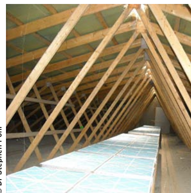
Figure 22 Filter box installed on a continuous linear air inlet
